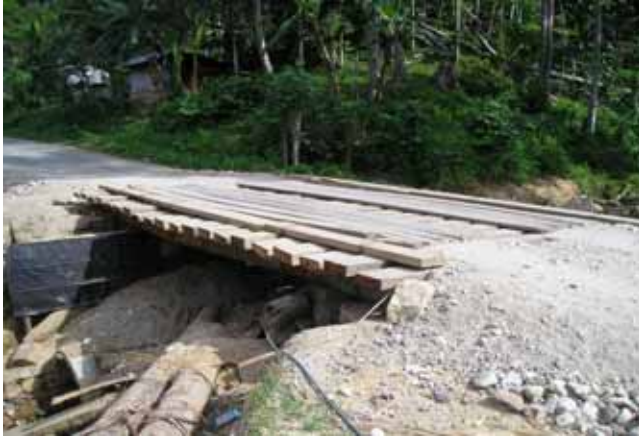
A temporary wooden bridge with maximum capacity 10 MT
