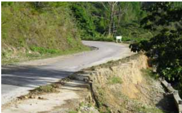
Slope stabilization under construction
