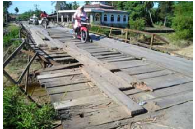
14.4 km north of Meulaboh, a new temporary bridge is being Constructed. Wooden Bridge, a bit damaged on the floor but still passable
