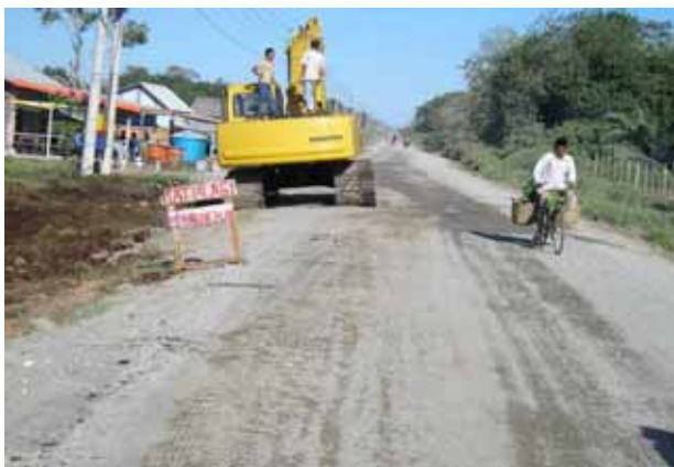
13 . 5 km north of Meulaboh , the road is already graded along 4.8km.
