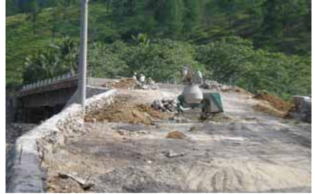
A new bridge under construction, almost completed
