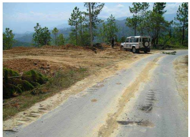
The road under construction for 100 m length
