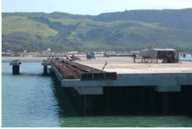
New Wharf at Port Malahayati
