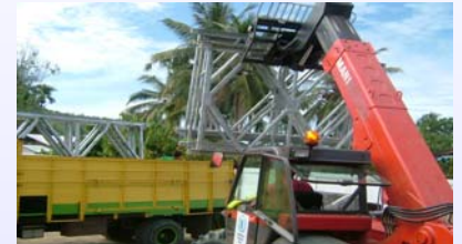
Manitou forklift unload part of Bailey bridge
